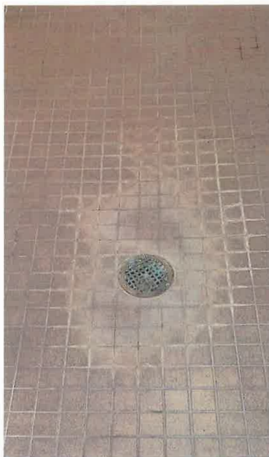
Shower drain repair caused by destabilization of slab
