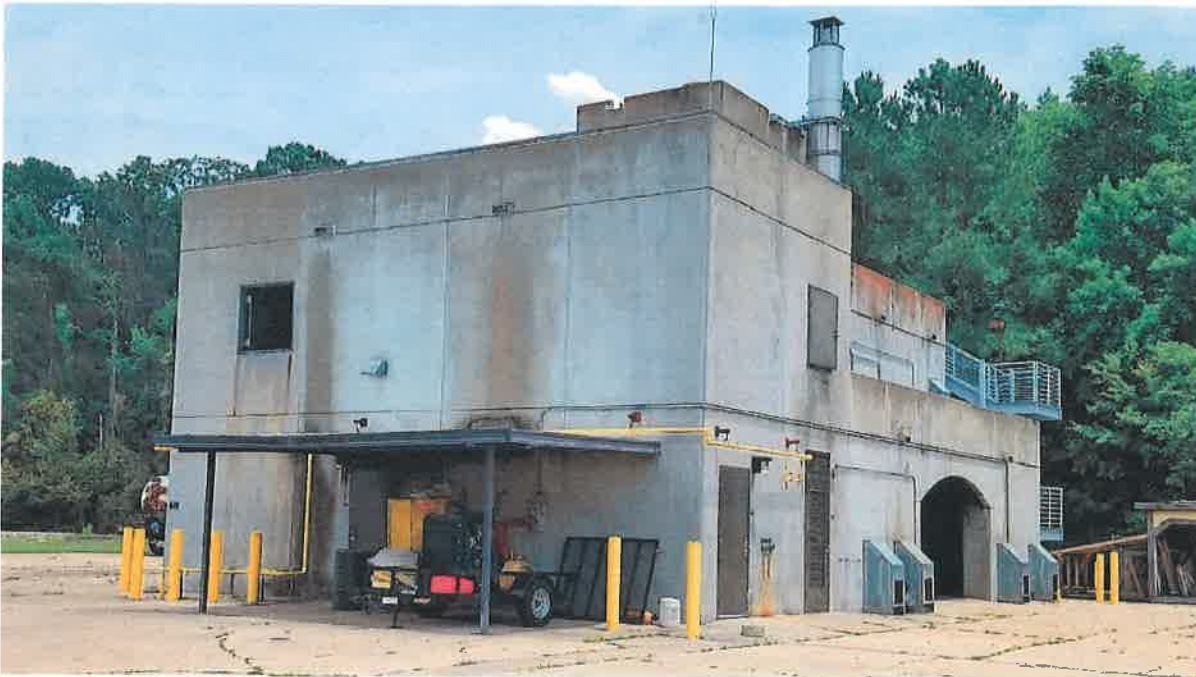
Burn Building, Building-W4
