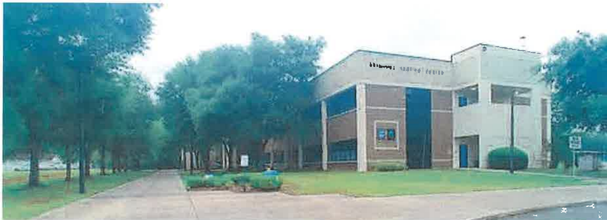
Criminal Justice Center, Building P, North Campus
